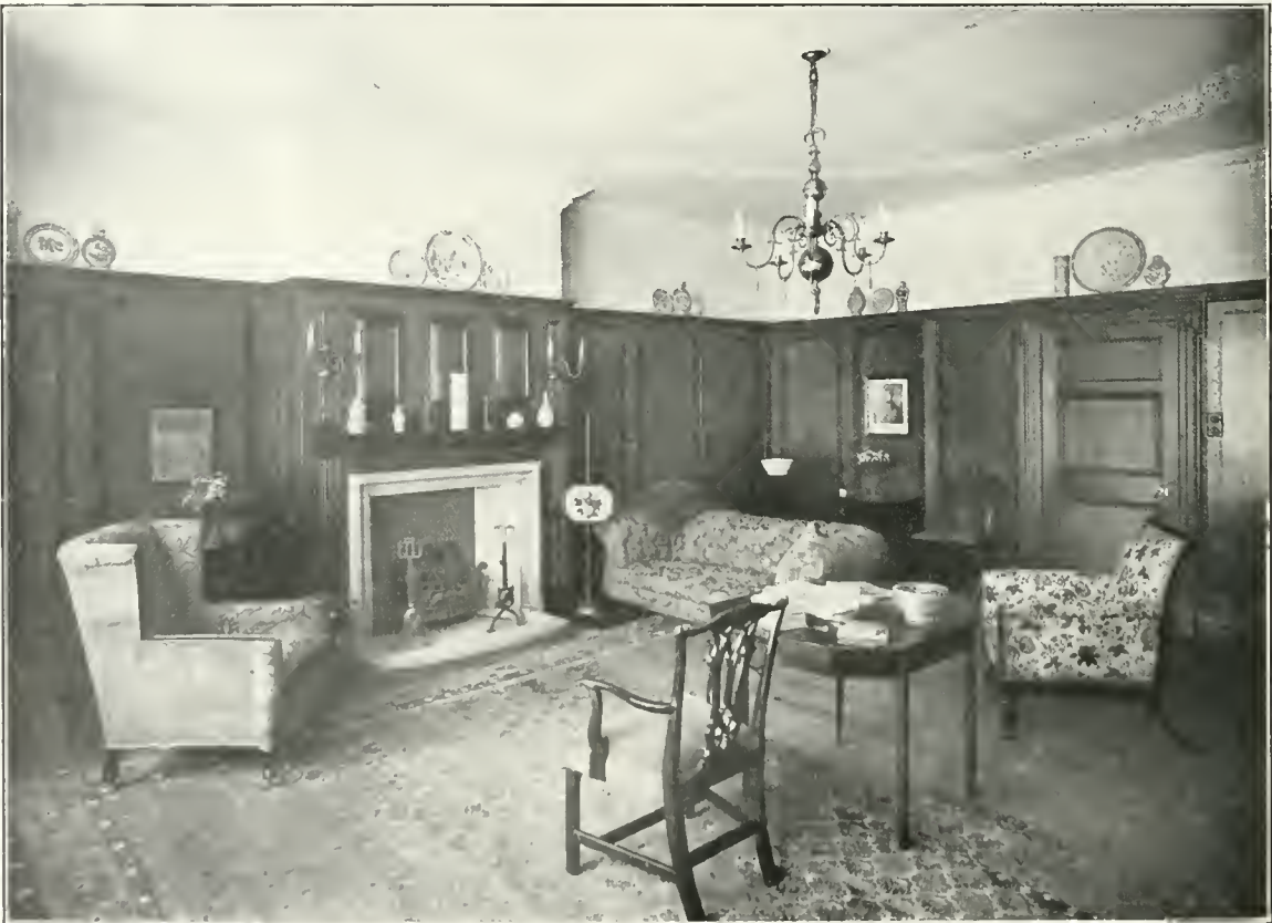
1. General view of new portion (west); the main front is to the south. 2. General view of the morning-room; the panelling is in fumed oak with mahogany inlay; modelled plaster ceiling.
